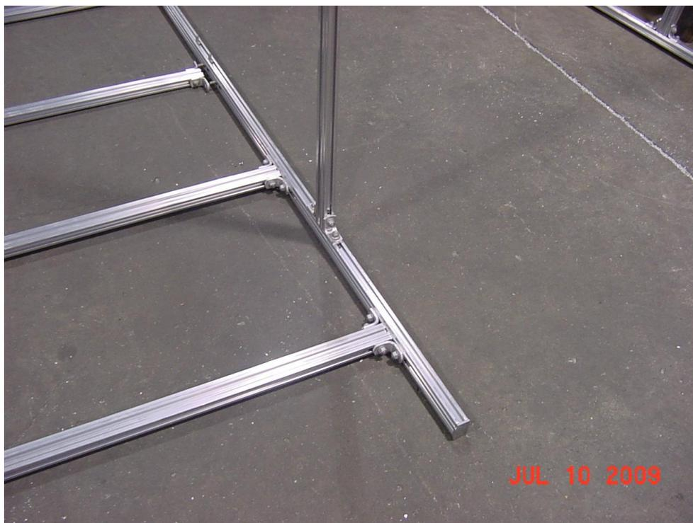
**Install the 4 cross bars that hold the two rack sections together on the “narrow” side of the uprights at the pencil marks.**
